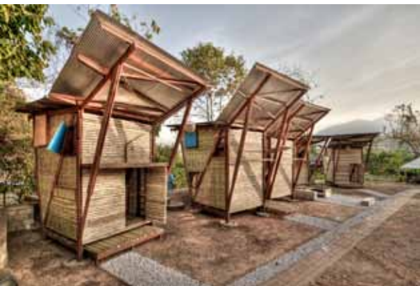
Architecture of Necessity Orphanage in Thailand. Tyin Tegnestue.
